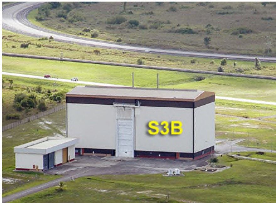
Figure 6.2.2.2.b – S3 area overview
